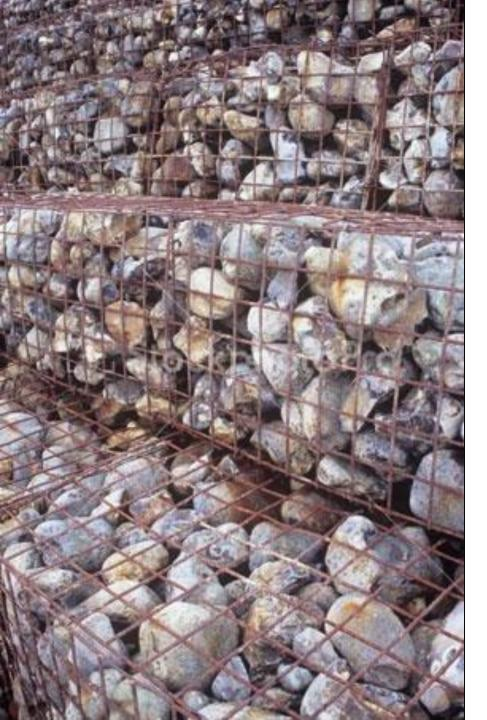
Gabions: wire cages filled with rocks. They are placed in front of cliffs, often stacked one on top of another, to **reduce erosion** and prevent cliff falls. They absorb the power of the incoming waves and prevent the cliff from slumping forwards.
