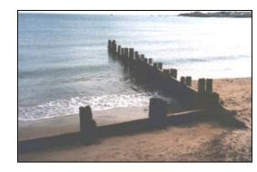
In 1991 a rock revetment and two rock groynes were built. Sand accumulated and halted erosion. • South of Mappleton, the rate of erosion has increased significantly. Material that usually moves south via longshore drift is becoming trapped within the groynes. Now there is no beach to protect the cliffs - the sea reaches the base of the soft
