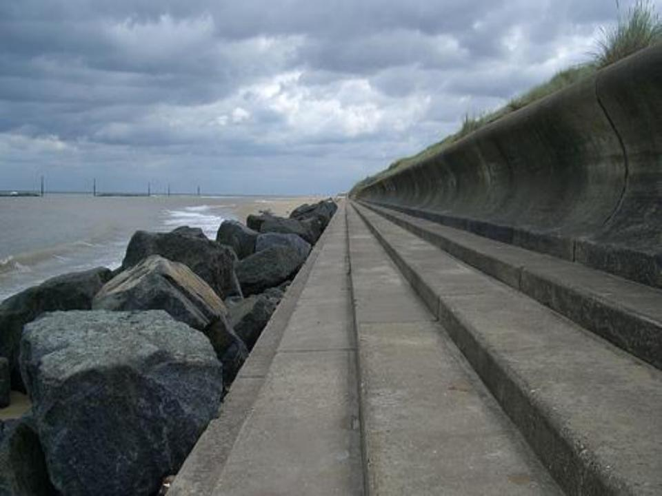
**Rock armour (rip-rap):** piles of large boulders are dumped at the **foot** of the cliff, or in front of a sea wall to reduce erosion by **absorbing the power** of the incoming waves. They also help prevent materials from being **scoured** from the beach by the backwash as the water is slowed down when it runs through the gaps between the rocks, reducing its power. Rock armour costs **£200,000 per 100m**.
