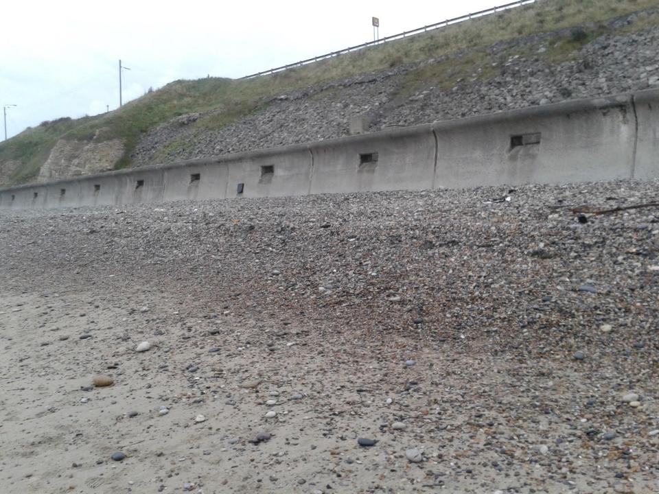
Sea walls are reinforced concrete structures that create a rigid barrier between the sea and the land. They are incredibly expensive to build - about £5000 per metre. Sea walls can be straight or have a curve at the top. This sends the energy of the waves back out to sea and is called splashback.
